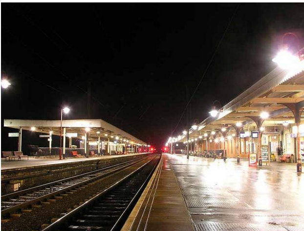
Access point - Ely railway station
